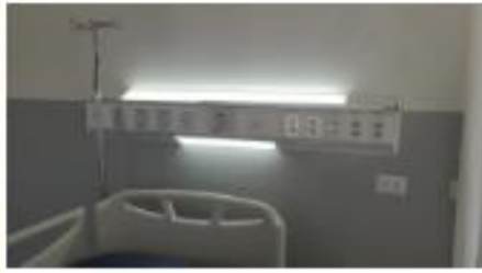
Panel with American outlets and a combination of American and Chilean sockets GCR model
