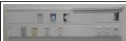
2 GCR channel panel with American outlets and Chilean and Schuko sockets
