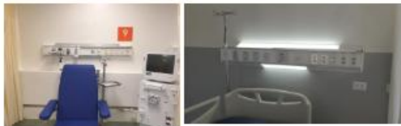
GCR Panel with American gases outlets and Chile / Brazil / Italy electric sockets
