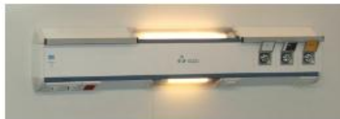
GCR Panel with AFNOR outlets and SCHUKO sockets.
